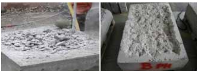
Figure 3. Pneumatic treatment (pick-hammering) of top concrete surfaces of blocks A and B
