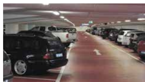
Figure 4. Parking spaces and lane with cars overlapping into the lane
