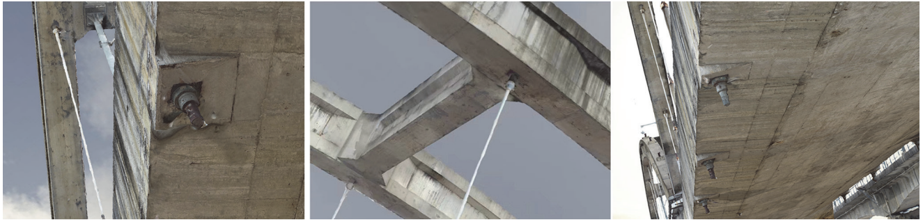
Figure 19. Details of bridge superstructure from below
