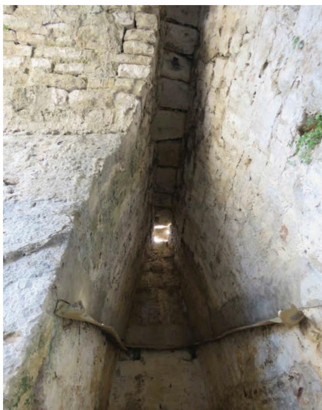
Figure 19. False ceiling at the S-W tower
