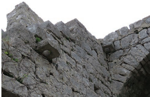
Figure 12. Perforated stone cantilevers – supports for the wooden railing (authors)
