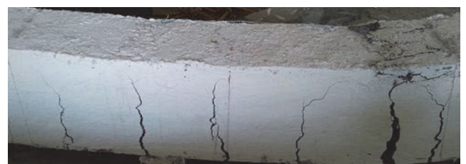
Figure 18. Crack pattern and failure mode of RC beam for copper slag 60% replacement and PP fibre 0,4 %
