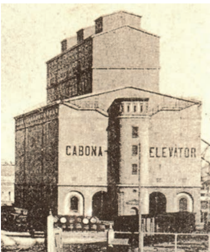
Figure 13. Grain silo, view on western front [26]
