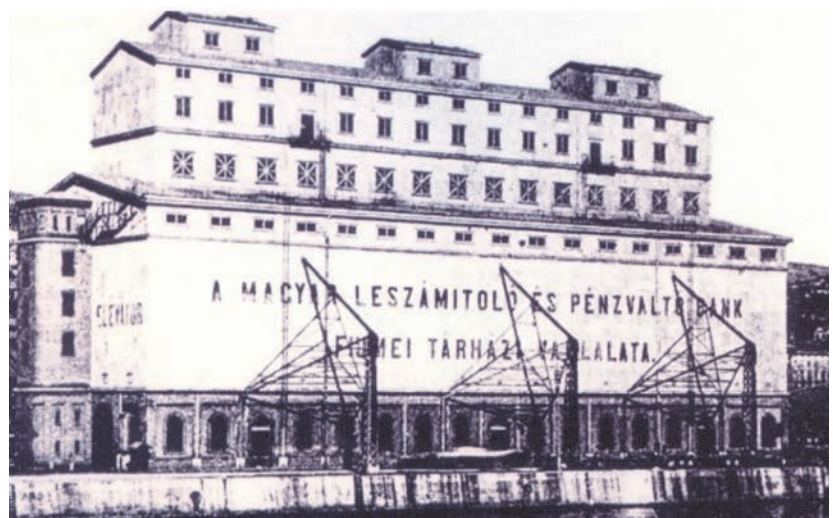
Figure 14. Grain silo, view on southern front [27]
